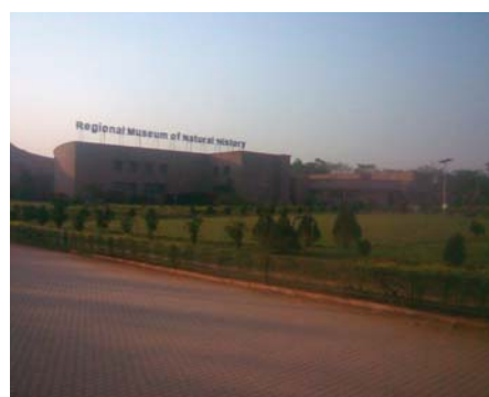
Rooftop solar project installations in Odisha
