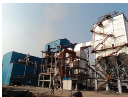
Rice Husk Power Plant
