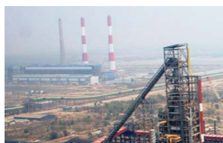
Coal Washery Power Project at Angul
