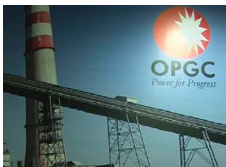
Two sub critical units of OPGC
