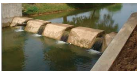
Diversion Weir, Khariar, Nuapada
